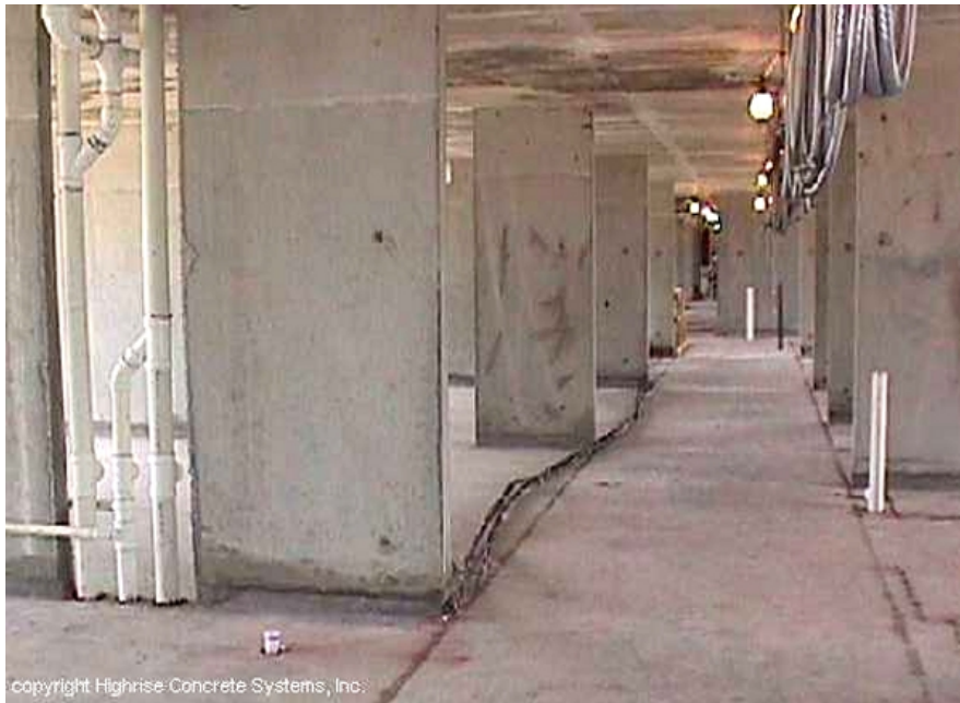
Figure 11 – an example of the results of blocked out tunnel form construction
